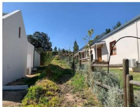
example of current post & rail with "Fortinet" wire in between rails
